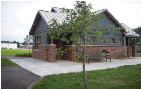
EXISTING RESTROOM BUILDING
