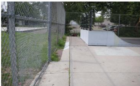
EXISTING SKATE PARK CONCRETE IS IN GOOD SHAPE
